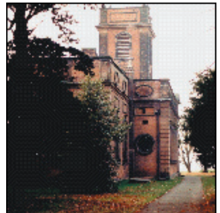
FIG 2: St Mary and St Margaret's Parish Church – Grade A Listed.
